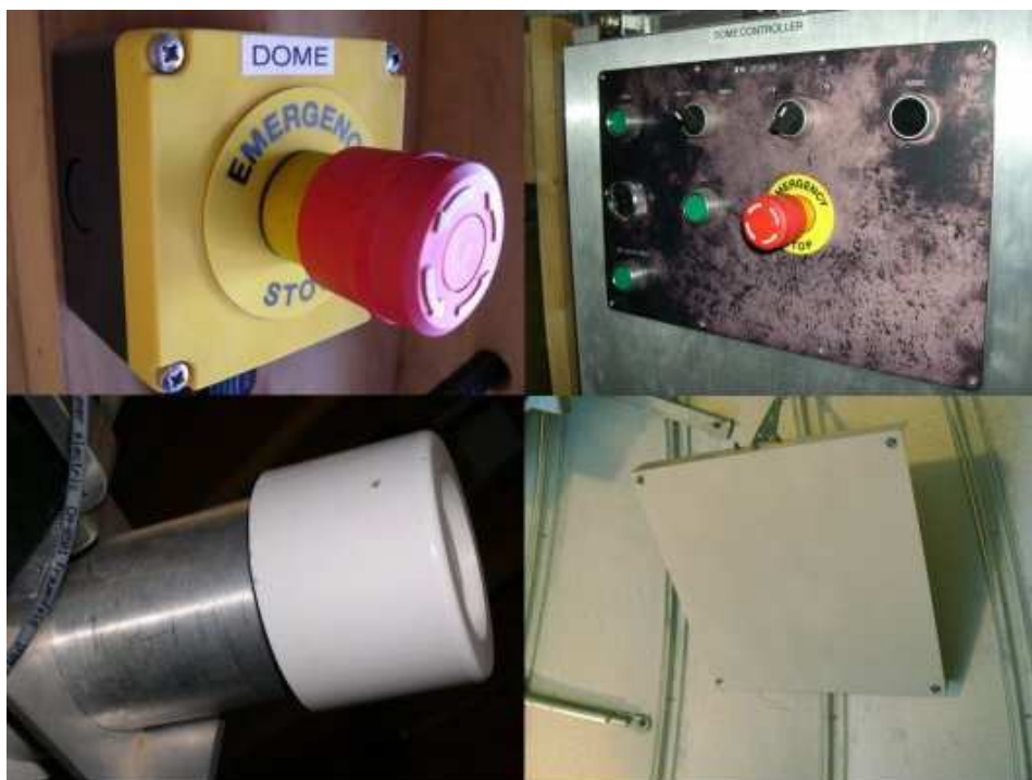
FIGURE 2.4— Different views of the STARE dome. From top left to bottom right: emergency stop button, dome control panel, flat-field lamp, flat-field screen.
